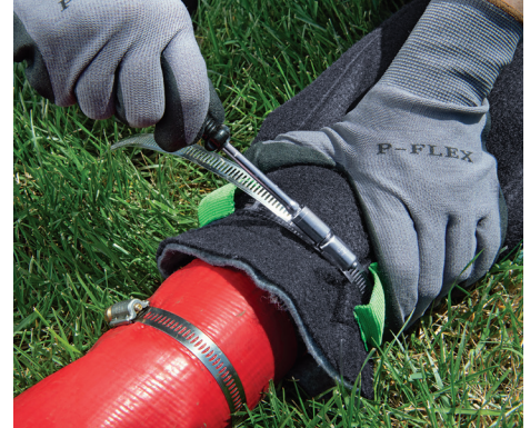
3. Fasten hose clamp tightly with a 5/16" nut driver.
