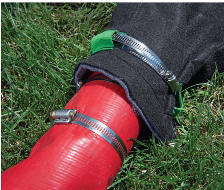
4. Tuck remaining hose clamp into green loops to secure.
