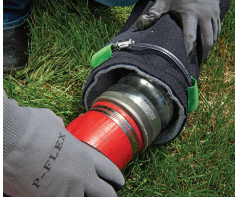
2. Place mouth of Pipe Filter Sock over discharge hose or pipe.
