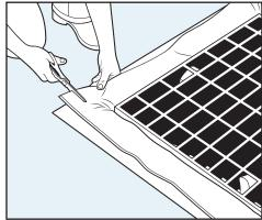
5. Remove tape and trim excess fabric, keeping roughly 7-8cm of material on all
