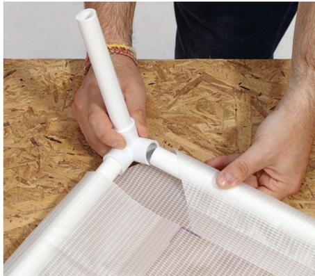
2. Slide the small support frame through the end pocket. Grasp the corner and insert the end of the support tube into the "Y" connector and snug into place. Repeat on opposite corner. Follow same steps for the other side of diverter.
